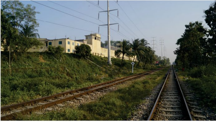
Illegal industry on hill, beside railway, sonaichori union.
