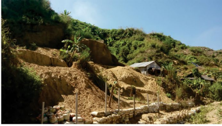
Hill cutting for informal settlement, salimpur union.
